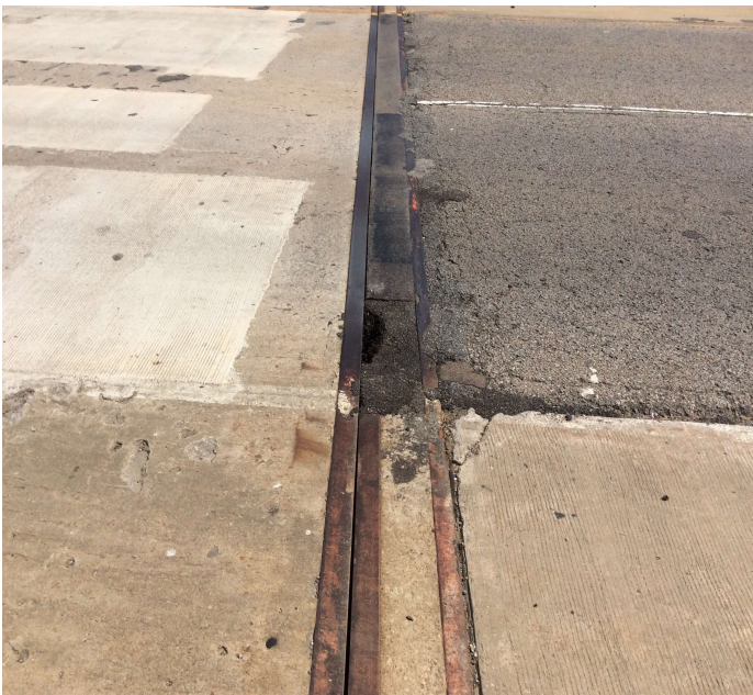
PHOTO 1 Description Bent 1 expansion joint
