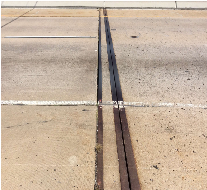
PHOTO 1 Description Bent 4 expansion joint
